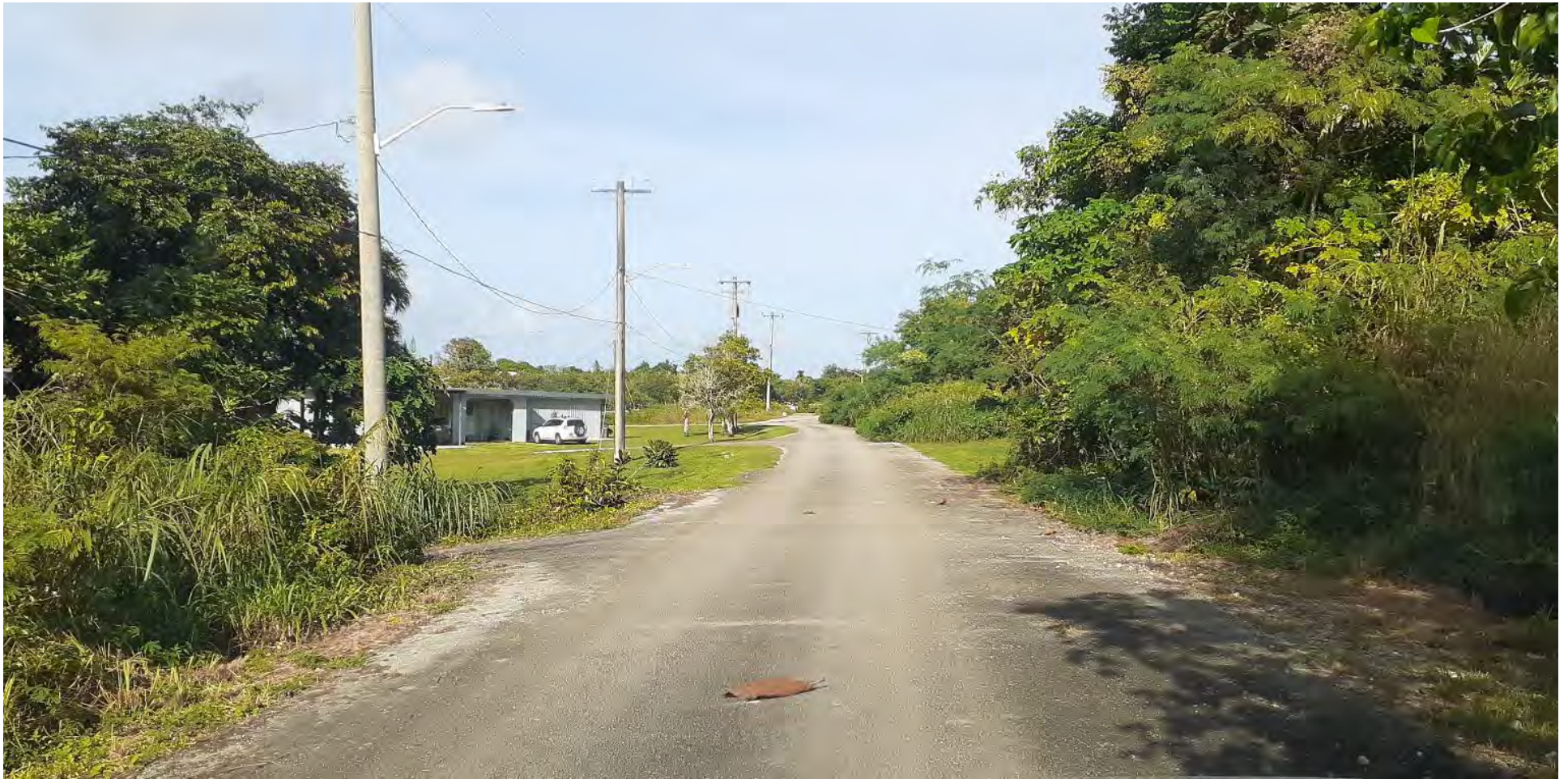
Photo 3. Golden Cupid Road within 1000 feet of well EX-11.
