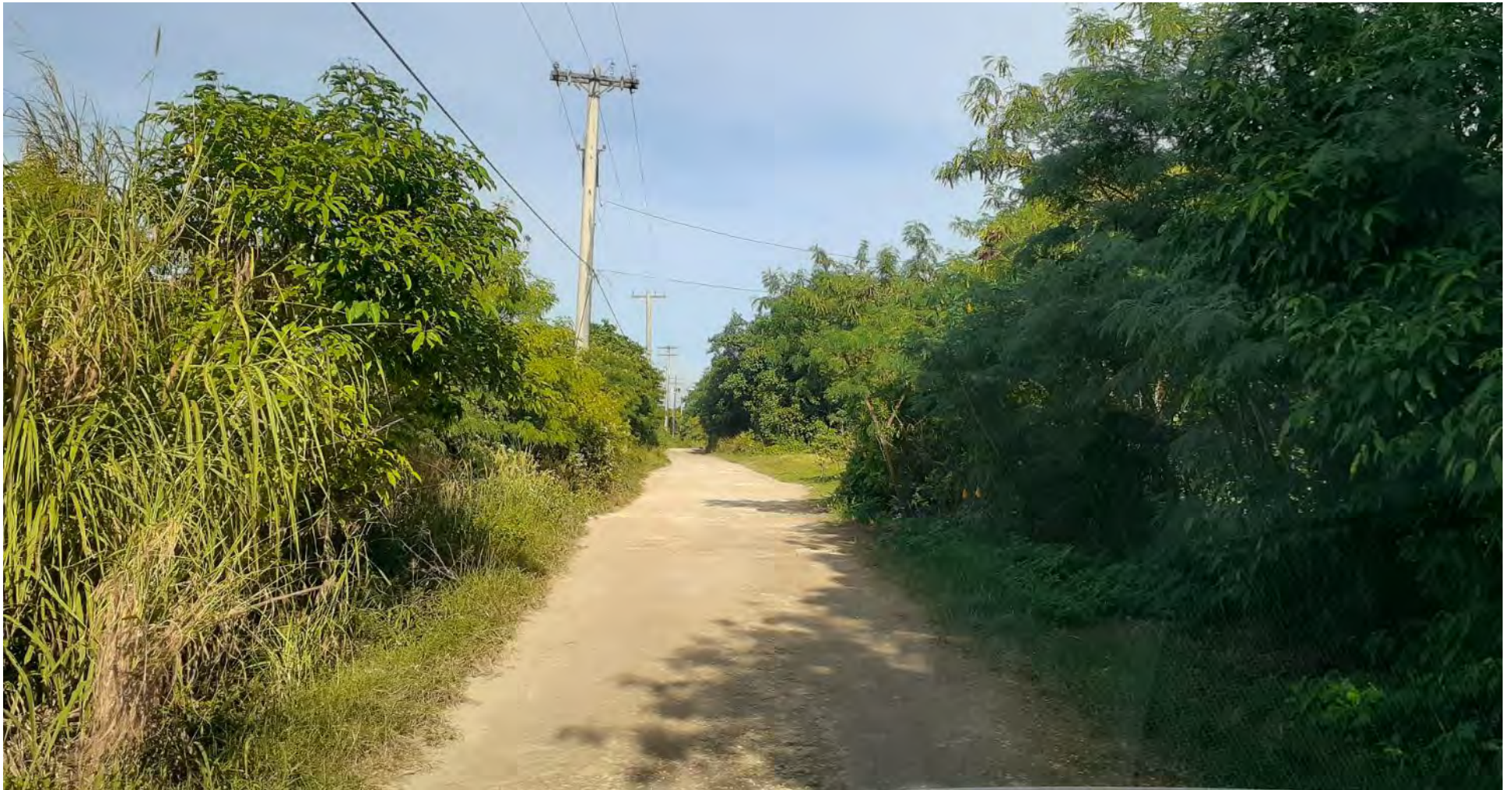
Photo 9. Road S-3 within 300 feet of well M-2.
